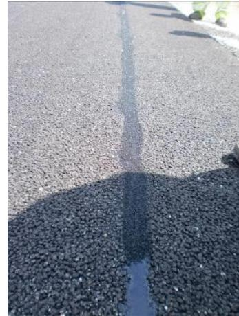
The masking tape applied to the sides of the repair area should be removed immediately after pouring and gritting. Approx. 60 minutes after application (at +23 °C/+73.4 °F), the compound is usually hardened to an extent where the road can be reopened to traffic.
