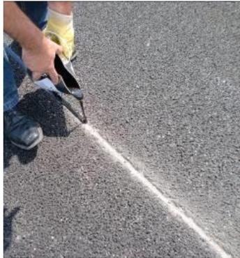
surface grip, it is necessary to sprinkle the compound with an excess of grit after it has been poured. For this, we recommend a grit with a PSV value (Polished Stone Value) of 40 to 60, grain size approx. 0/5. It is vital to ensure that the grit is dry when applied.
